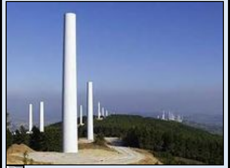
Fig 8(a) Tubular tower
